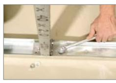
10. Tighten the M12 nuts on the anchors **H** at the top and bottom (torque 60 Nm).
