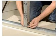
Position the four deformation brackets E, each with the undulating side pointing towards the UA profile K at its upper and lower end, align the UA profile K and mark the anchor holes on the unfinished ceiling and floor (see Overview 3.1).
