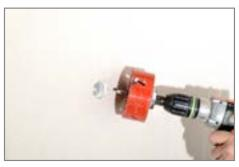
14. Align the hole cutter with 6 mm guide drill with the central hole of the absorber B and cut out the hole from the ceiling cladding. When doing so, do not cut into the cladding layer(s) underneath. Remove the round cut-out and level out the wall/attachment shell.
