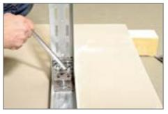
Insert 2 screws I each at the top and bottom on the UA profile K and secure the deformation brackets E using the counterplates F with the maximum permitted torque (27 Nm).
