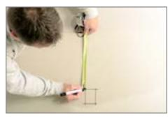
11. Prepare the first plate position, calibrate and mark the position of the absorber **B**.
