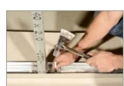
6. Clean the drilled holes and position the anchor **H** (FAZ M12).
