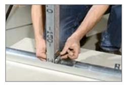
Insert the deformation brackets E (see Overview 3.1) and loosely tighten M12 nuts of the concrete anchors
