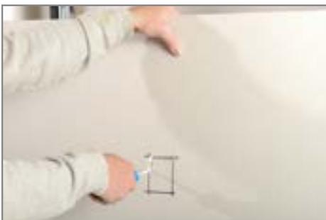
12. The opening for the absorber **B** is cut out in the first plate position using a keyhole saw in a rectangle of approx. 70 x 45 mm, meaning that the first plate position is solidly on the substructure and can be secured. The absorber **B** sits flush with the reverse of the relevant ceiling cladding.
