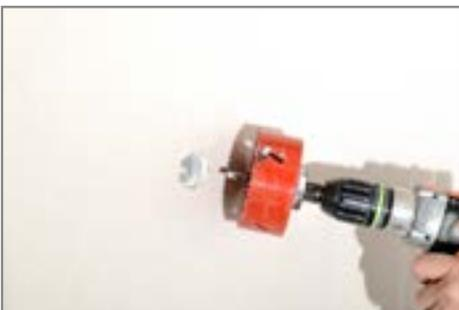
14. Align the hole cutter with 6 mm guide drill with the central hole of the absorber **B** and cut out the hole from the ceiling cladding. When doing so, do not cut into the cladding layer(s) underneath. Remove the round cut-out and level out the wall/attachment shell.
