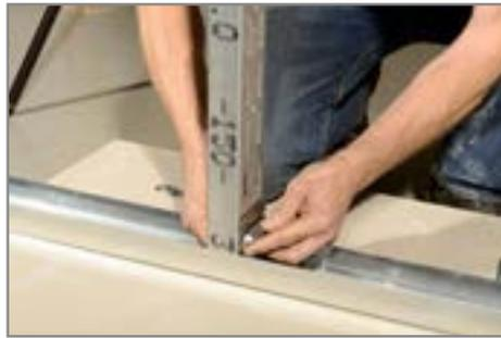
4. Position the four deformation brackets **E**, each with the undulating side pointing towards the UA profile **K** at its upper and lower end, align the UA profile **K** and mark the anchor holes on the unfinished ceiling and floor (see Overview 3.1).
