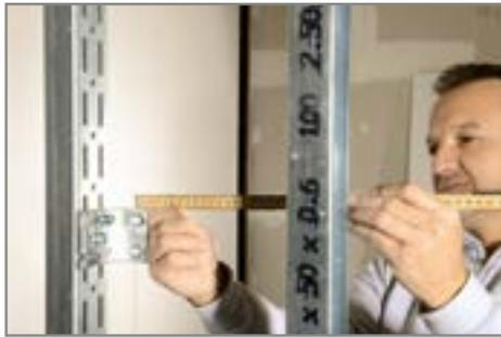
3. Push the UA profile **K** into the UW connection profile on the ceiling and unfinished floor and align to be precisely perpendicular with the back of the profile 30 mm to the right of the position of the anchor point **A** according to the plan.
