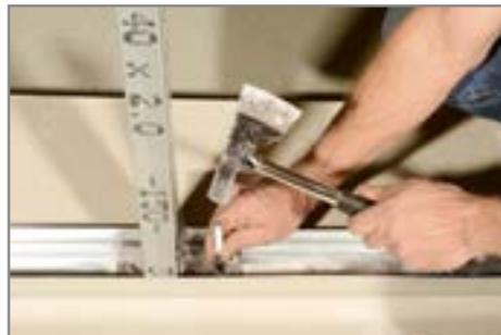
6. Clean the drilled holes and position the anchor **H** (FAZ M12).
