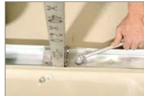
10. Tighten the M12 nuts on the anchors **H** at the top and bottom (torque 60 Nm).
