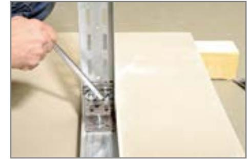
9. Insert 2 screws **I** each at the top and bottom on the UA profile **K** and secure the deformation brackets **E** using the counterplates **F** with the maximum permitted torque (27 Nm).
