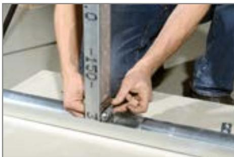
7. Insert the deformation brackets **E** (see Overview 3.1) and loosely tighten M12 nuts of the concrete anchors **H**. This means that the deformation brackets **E** can still easily be aligned to the UA profile **K**.
