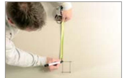
11. Prepare the first plate position, calibrate and mark the position of the absorber **B**.
