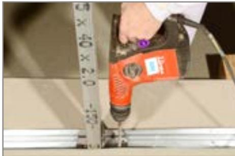
5. Drill two anchor holes each in the unfinished ceiling and floor to a depth of 110 mm.
