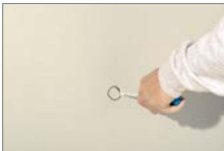
13. Adjust the relevant ceiling cladding, calibrate the centre of the absorber **B** (central 6 mm hole) to the correct position and mark as precisely as possible on the prepared plate. Cut out a roughly coin-sized opening at the marked position. Secure the ceiling cladding to the substructure.
