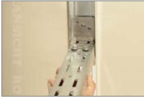
3. Screw on two deformation brackets **E** back to back on the UA profile **J** with two M8 screws **H** and a counterplate **F** (do not fully tighten the screws at this point).
