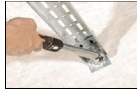
8. Tighten M8 screws **H** on the top and bottom (tightening torque 27 Nm).
