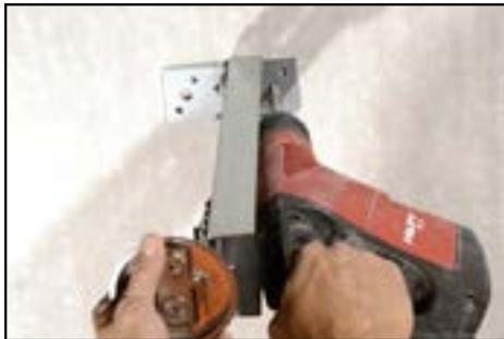
5. Mark holes for screw holes on the ceiling and drill 2 x 12 mm holes to a depth of 110 mm.
