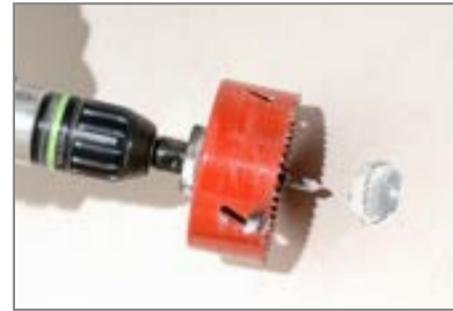
9. Adjust the ceiling cladding or acoustic plate, calibrate the central point of the absorber **B** and cut out an opening with a hole cutter.
