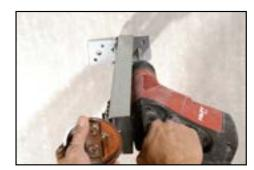
Mark holes for screw holes on the ceiling and drill 2 x 12 mm holes to a depth of 110 mm.
