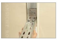
Screw on two deformation brackets E back to back on the UA profile J with two M8 screws H and a counterplate F (do not fully tighten the screws at this point).
