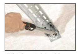
8. Tighten M8 screws **H** on the top and bottom (tightening torque 27 Nm).
