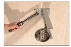
6 Secure 2 deformation brackets E with the attached UA profile J to the load-bearing structure using 2 x Fischer FAZ M12 anchors G (tightening torque 60 Nm). Clean the drilled holes and position the anchor G (FAZ M12).
