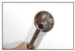
10. Completion: Secure socket C and anchor point A with 2 countersunk screws D. When doing so, the "front side" marking on the buckle must be visible. If necessary, correct the position of the absorber B so that the socket C is flush with the soffit (visual inspection).
